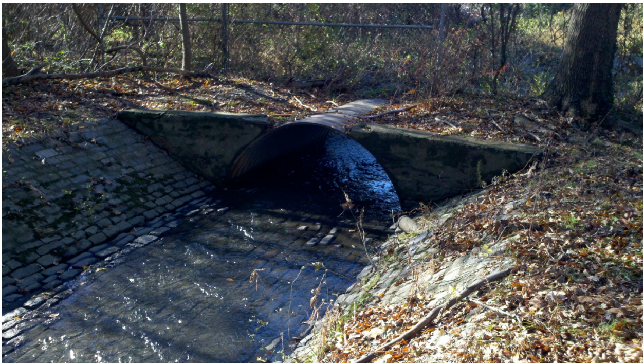
Photo 2: Malbone Channel - Looking west at culvert approx. mid-point of channel.
