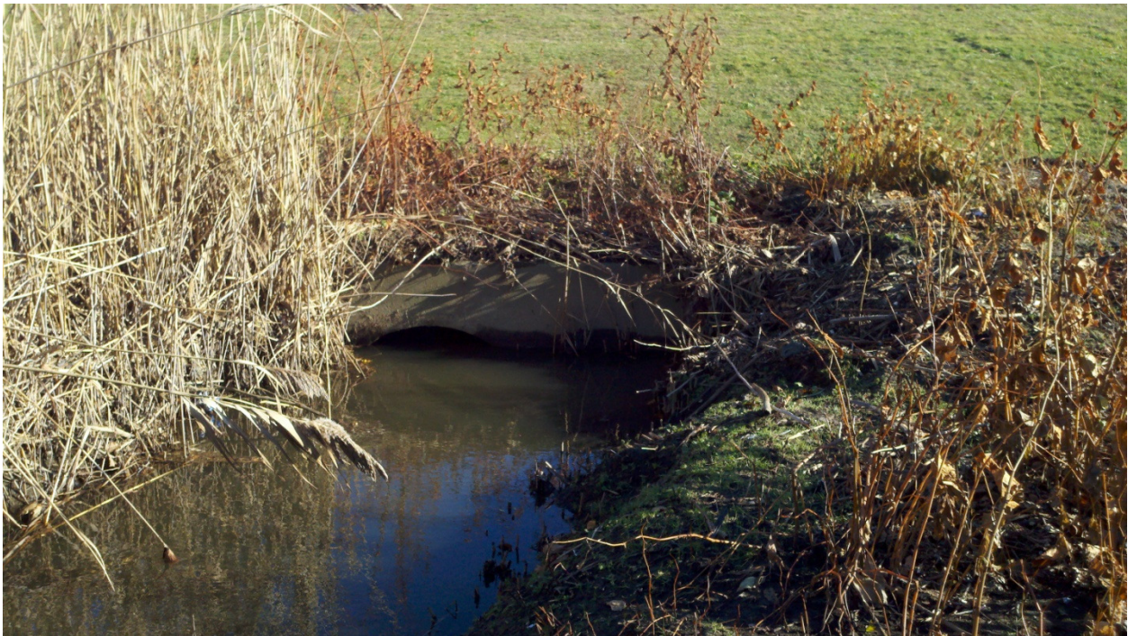
Photo 4: Outlet of Double-Barrel Culvert under RI 138/138A/238 - Looking east from rear of 111 JT Connell Road.
