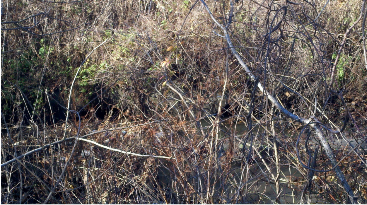
Photo 3: Double-Barrel Culvert under RI 138/138A/238 – Looking west at City Drainage Swale from rear of DPW Yard.
