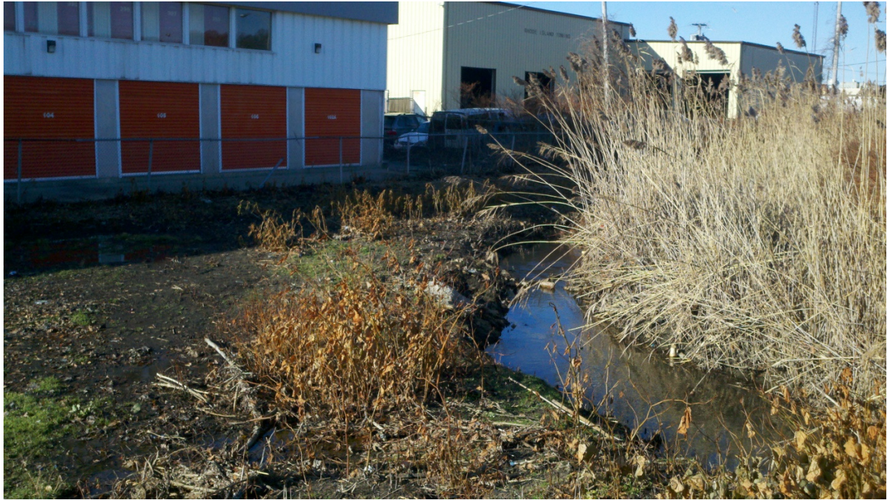
Photo 5: Drainage swale at rear of 111 JT Connell Rd. - Looking north towards rotary.
