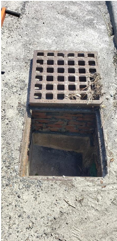
Photos 8, 9, 10. Existing Condition of Drainage Catch Basin and Manhole on Bellevue Avenue near Reject's Beach and Cliff Walk Entrance, CB-193-150 and DMH-193-151
