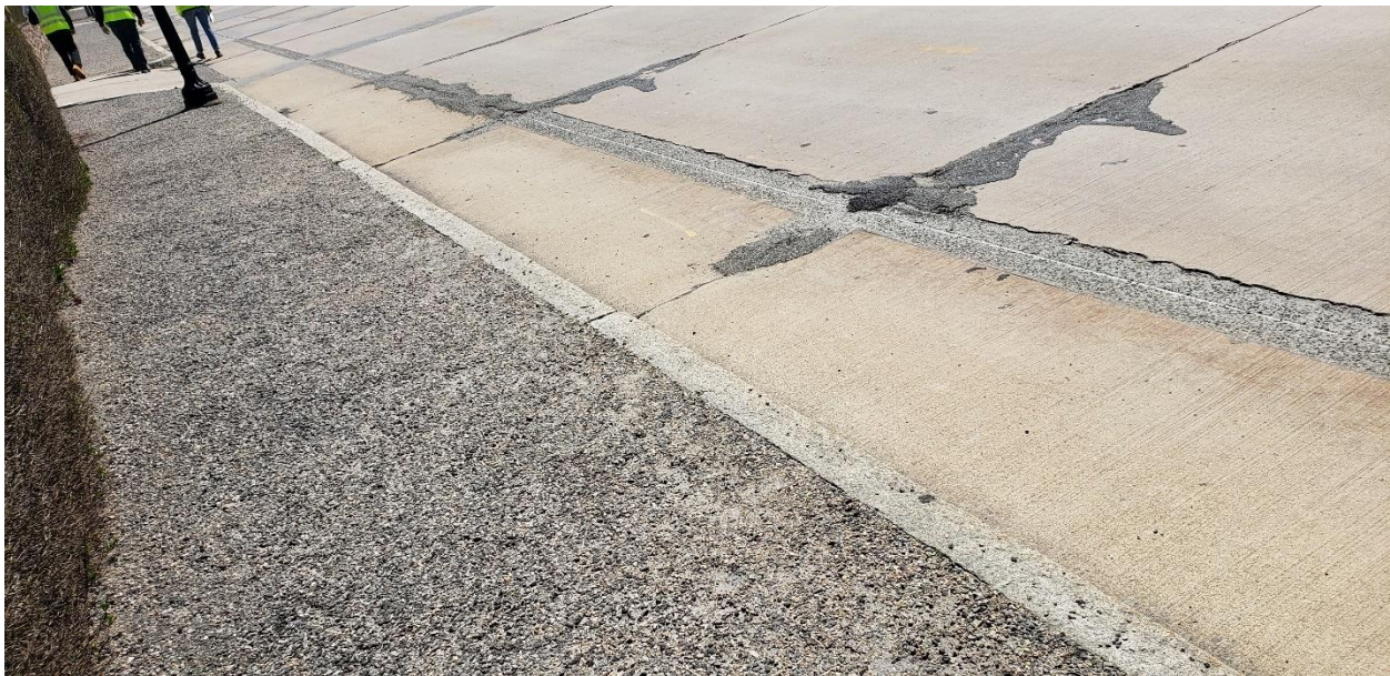
Photo 6. Existing Condition of Crushed Bluestone Sidewalk on Bellevue Avenue Photo taken April 2023
