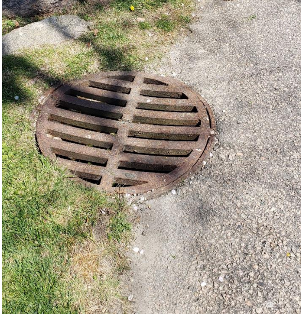
Photo 11. Existing Condition of Drainage Catch Basin on Ledge Rd, CB-194-161
