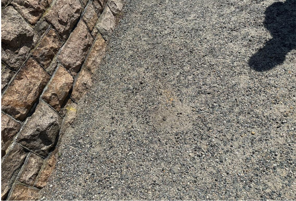
Photo 7. Existing Condition of Crushed Bluestone Sidewalk on Bellevue Avenue
