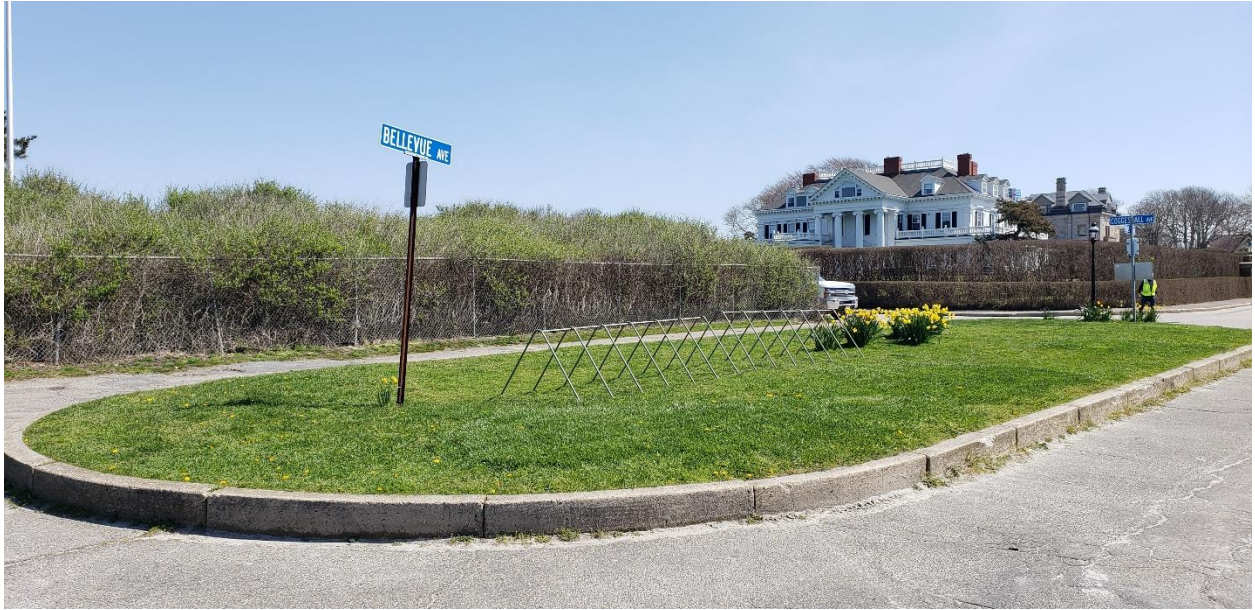
Photo 3. Existing Grass Median at Intersection of Bellevue Avenue and Coggeshall Avenue Photo taken April 2023
