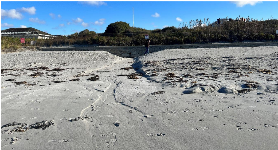
Photo 2. Existing Storm Outfall at Rejects Beach, DO-193-1
