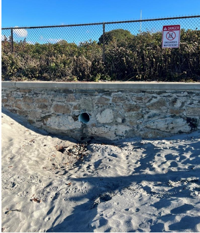
Photo 1. Existing Storm Outfall at Rejects Beach, DO-193-1
