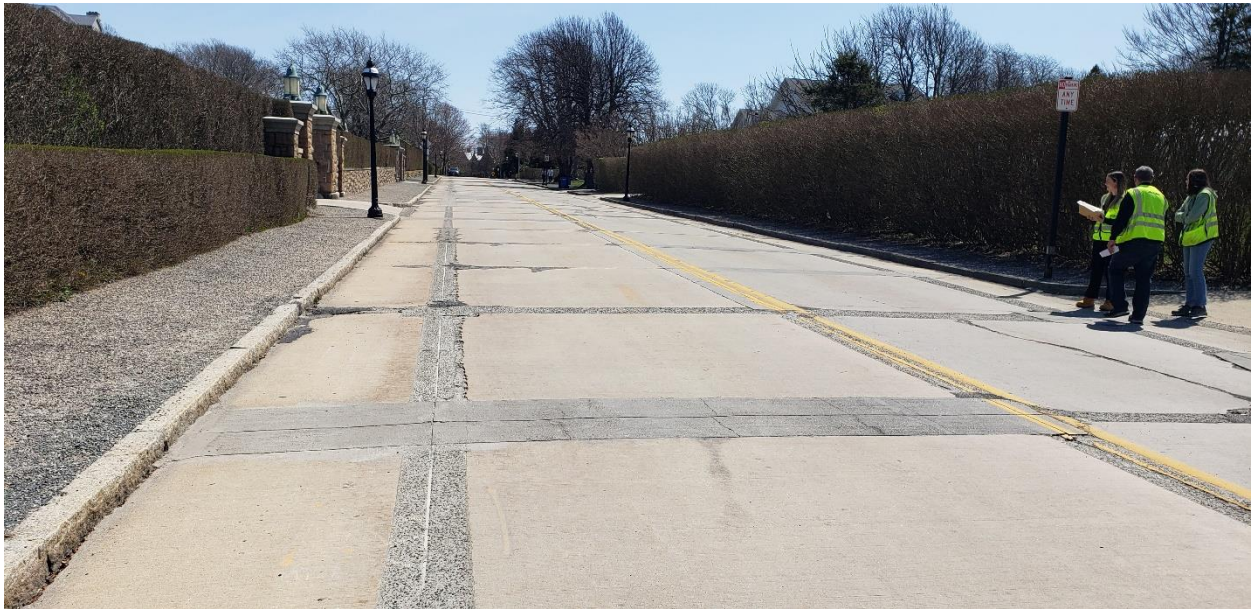
Photo 4. Existing Condition of Bellevue Avenue, Looking East Towards Ledge Road Photo taken April 2023
