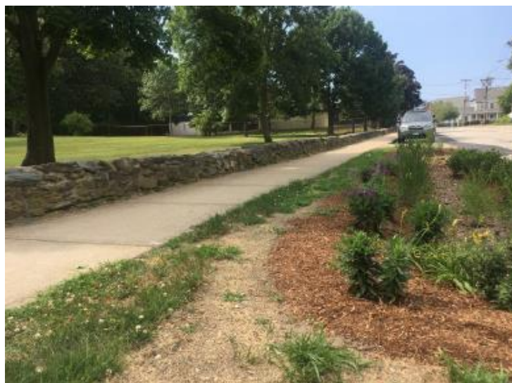
Figure 3-2. Hillside Avenue Installed Bioretention Area
